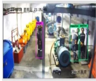
Underground staff monitoring
